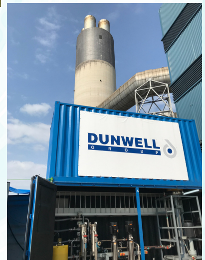
Power plant waste washing acid treatment
