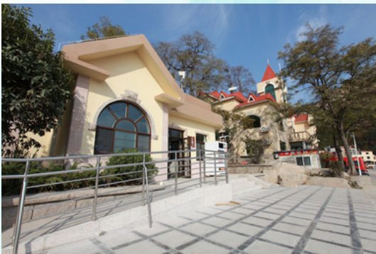
Bio-Toilet municipal wastewater treatment and reuse in Laoshan Tourist Area
